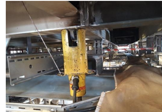
Davit Arm Load Testing
