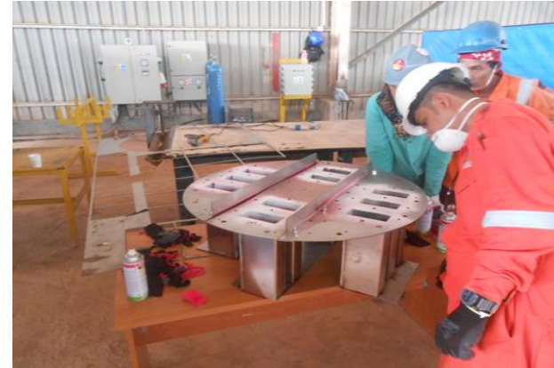
Dye Penetrant Test
