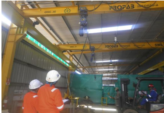
Overhead Crane Inspection
